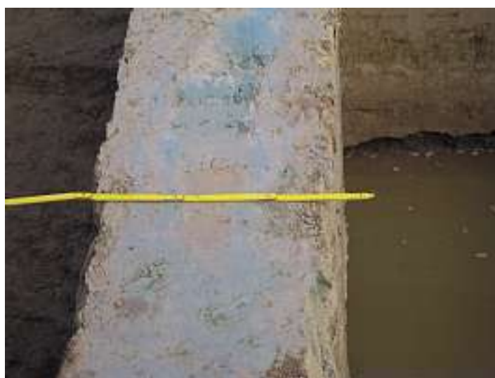
Figure 2.13: Sample of the finished MIP wall
