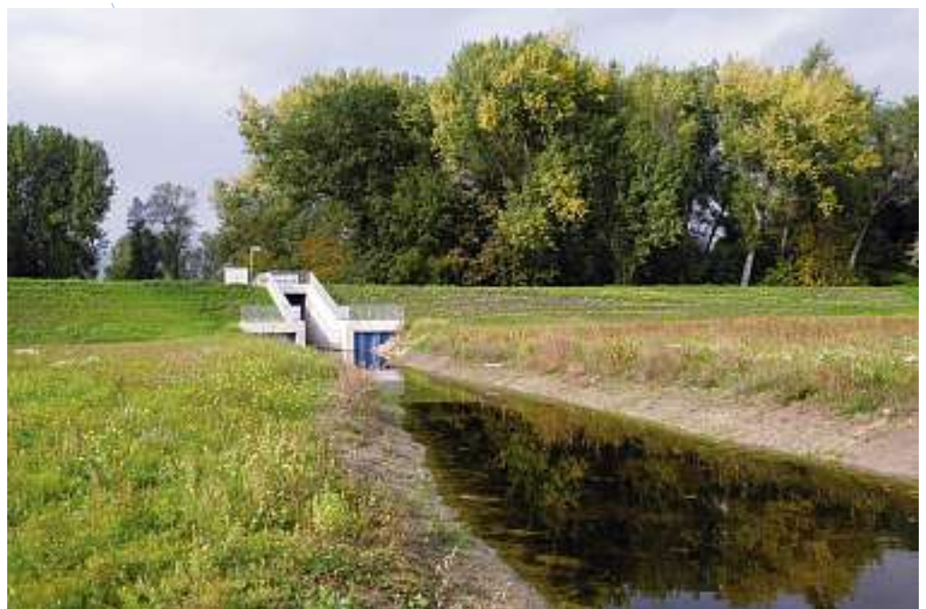
Figure 3.16: Inlet structure ecological flooding
