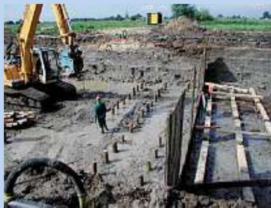
Figure 2.67: Wooden pile foundations of the culverts (inlet works)
