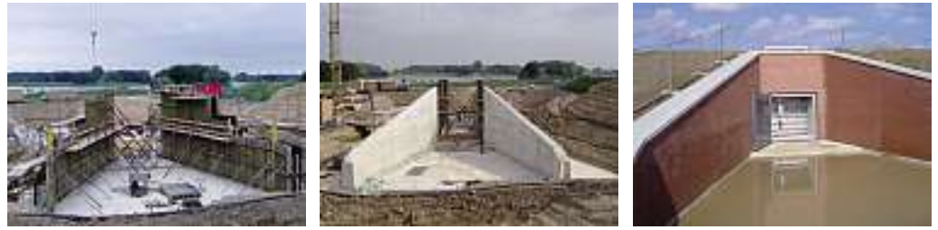
Figure 2.24: Inlet structure, return walls (left to right): formwork, concrete, clinker layer
