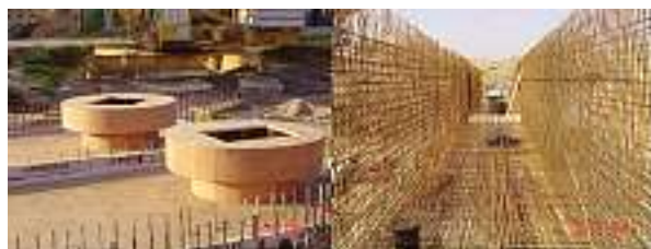
Figure 2.54: Lohrwardt Polder pumping station, formwork November 2005 and reinforcement passage June 2005
