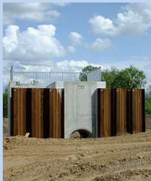
Figure 2.48: Culvert Dike East under construction with incorporated sheet pile walls
