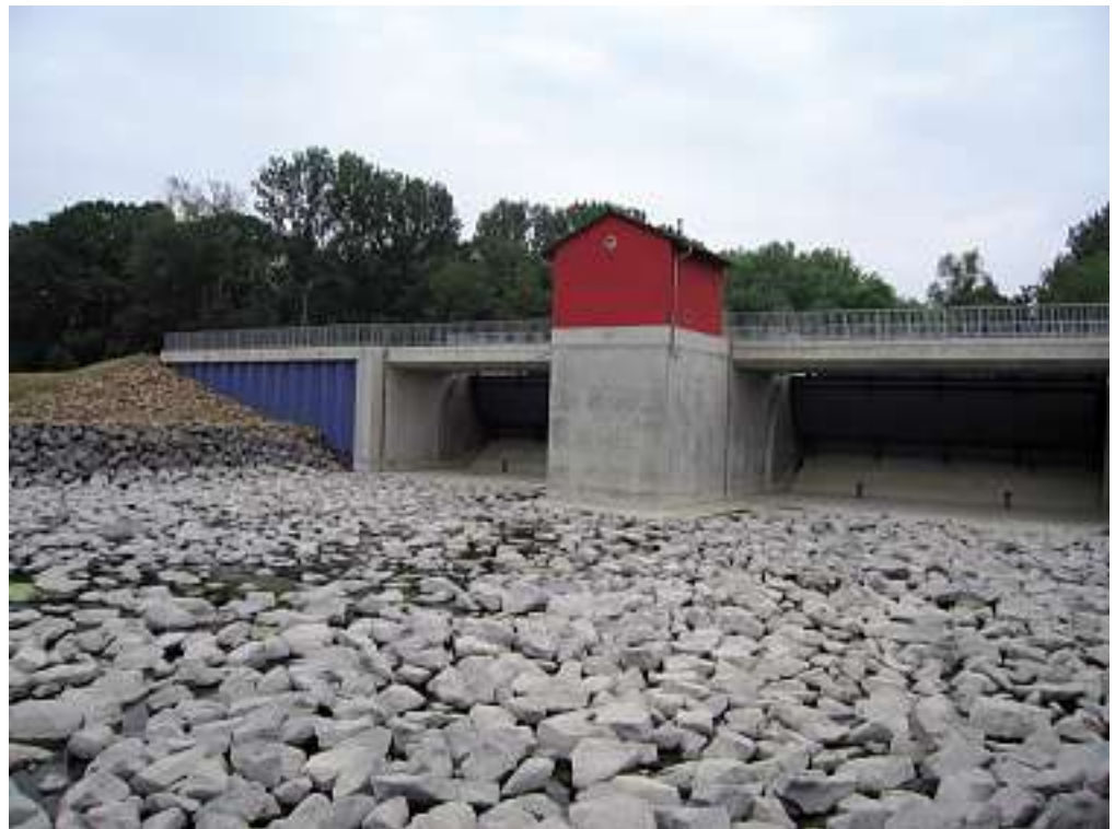
Figure 2.29: Stilling basin Ingelheim Polder – ready for operation
