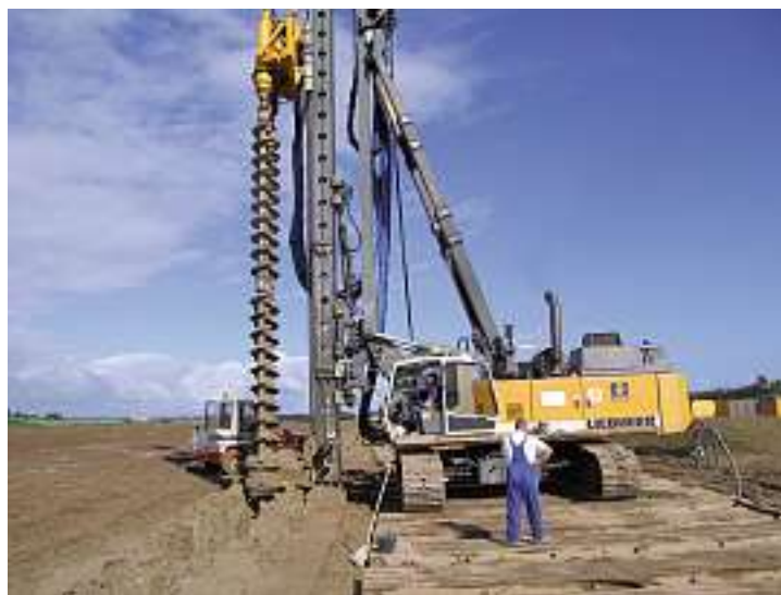
Figure 2.11: Construction of the MIP cut-off wall
