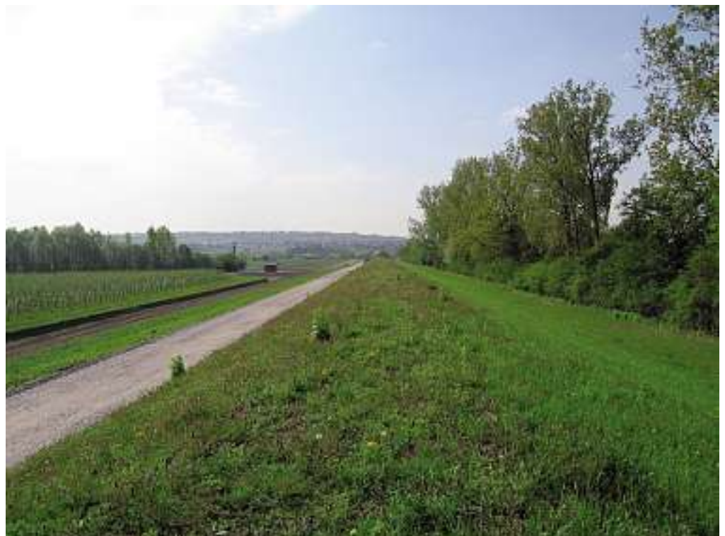
Figure 3.7: Sowing of the new dikes by means of the Heudrusch procedure
