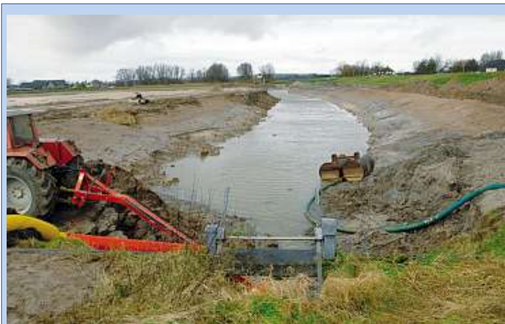
Figure 2.58: Hondsbroeksche Pleij seepage ditch construction
