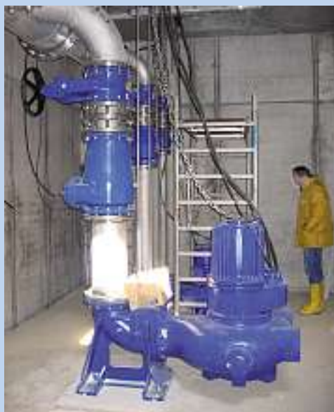
Figure 2.47: Underground portion of the pumping station with submersible pumps
