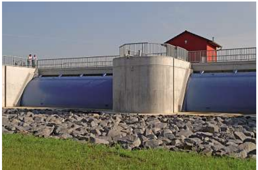
Figure 2.19: Inlet structure Ingelheim Polder, view from riverside.
